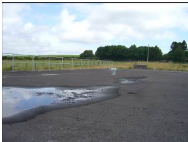
Plate 12.2: Water Reservoir at Moneygourney
