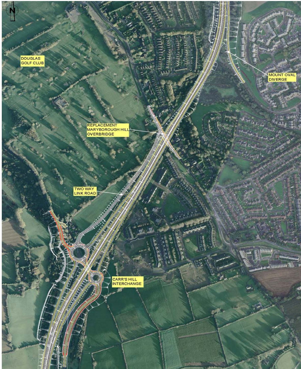
Figure 4.11: Carr's Hill Interchange – April 2016
